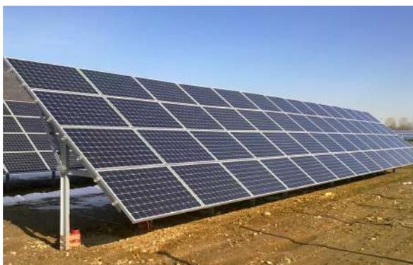
🇬🇧 A ground installation is a photovoltaic system positioned on the ground. It has the same functions and components as a classical system but it can provide two types of service.
